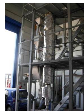
Fig. 3. Gasification unit in Greece.
