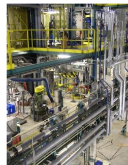
Figure 5: Arkema pilot plant equipped with a 100 L reactor.
